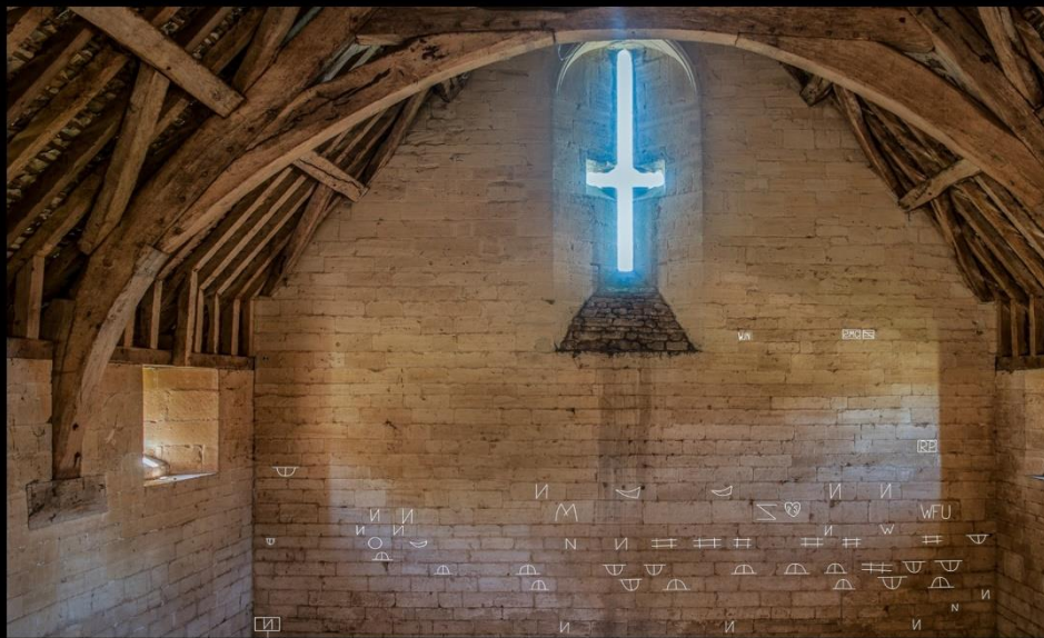
Plate 18: West Wall interior. Large number of mason's marks (annotated above actual size(, particularly when compared against east wall which has none. Possible rebuild on East wall?
