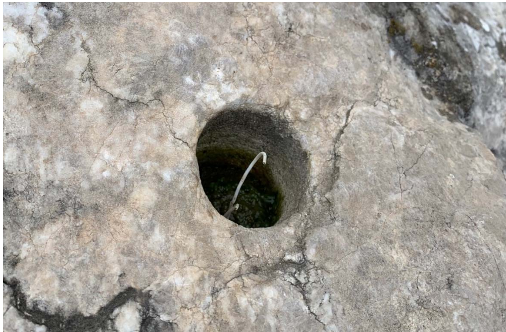
Fig. 8: Evidence of dynamite usage in the damage of the southwest corner of the monument. Photo by Author.
