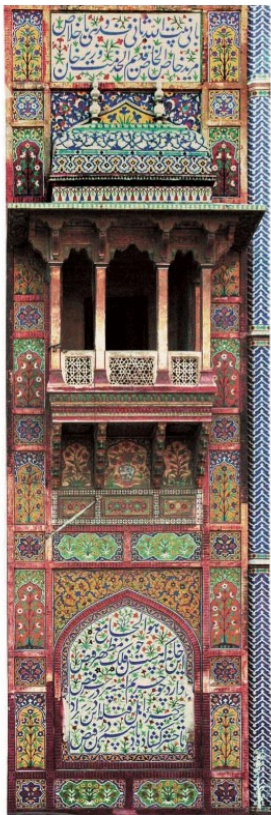
Fig. 6. Fresco work, tile inlay work and faux brickwork on the main portal of the mosque. (Source: AKCSP )
